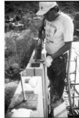
Post tensioning of CMU system
