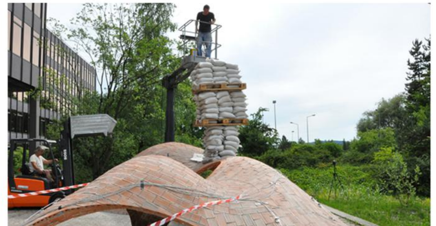
Load Testing with Sandbags
